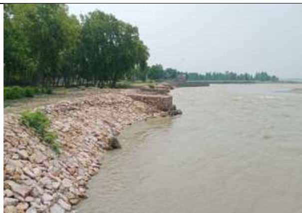
Gabion Wall Works at Dhaggi Faizaulah (Package 11)
