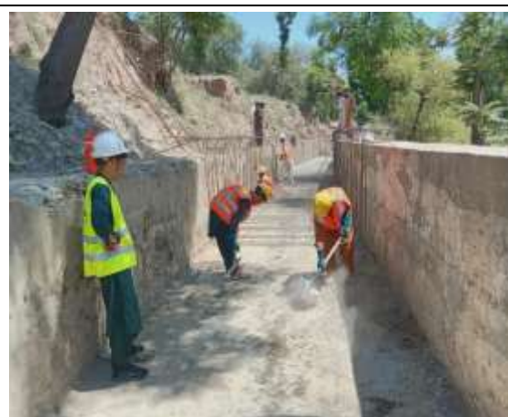
Workers working in the Irrigation Channel
