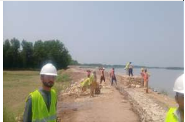
Construction Activities with PPEs and Limited Safety measures at Package 6 (Reach 2)
