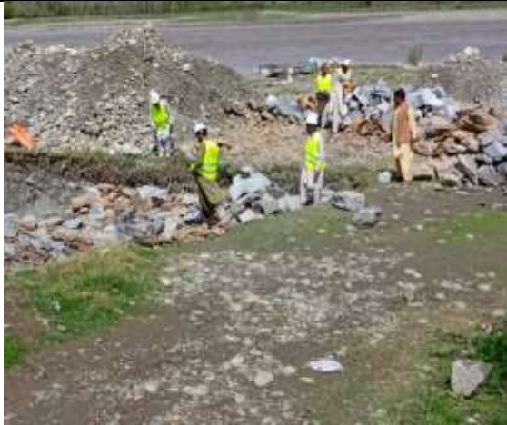
Gabion Wall Caging in progress
