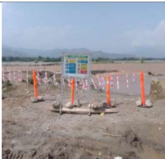
Barricading and safety signage (Package 14, Bandkurai and Ketch Minor)
