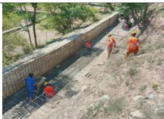
Construction Activities with PPEs and Limited Safety measures at Dir
