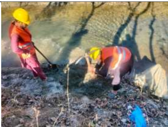
Cleaning work in progress
