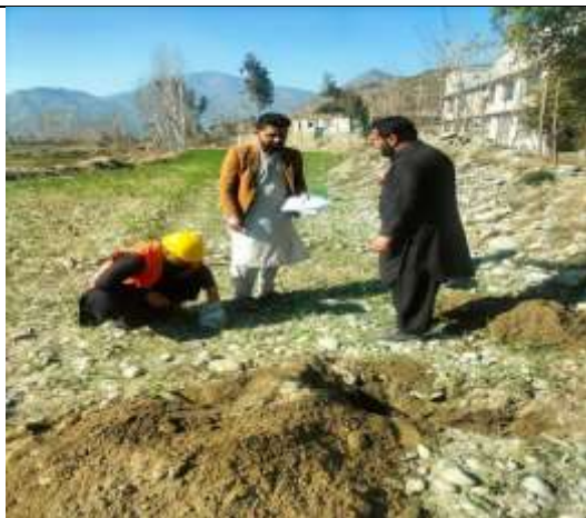
Soil Investigation at site
